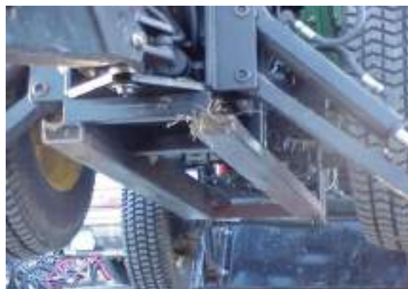
Figure 43. Hoe frame reinforcement after view
