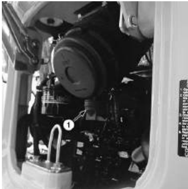
Air Cleaner Dust Unloader Valve
