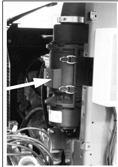
Figure 5.2 Intake air filter of the engine
