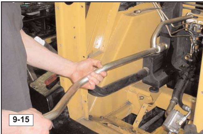
15. Disconnect the main oil cooler line from the junction block, then remove it from the machine. (fig. 9-14, 9-15)
