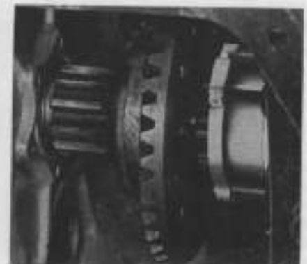
Fig. MH366—Removing differential bearing caps using OTC tool MH670 on models 201, 202, 203, 203G and early 55 & 55K models.
