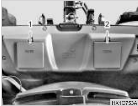
(1) Fuse Box 1 (2) Fuse Box 2
