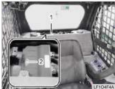
(1) MCU (Machine Control Unit) (2) Lamp
