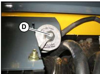
Figure 42 – Battery Disconnect Switch
