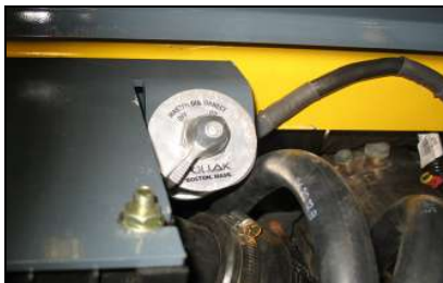
Figure 14 – Battery Disconnect Switch
